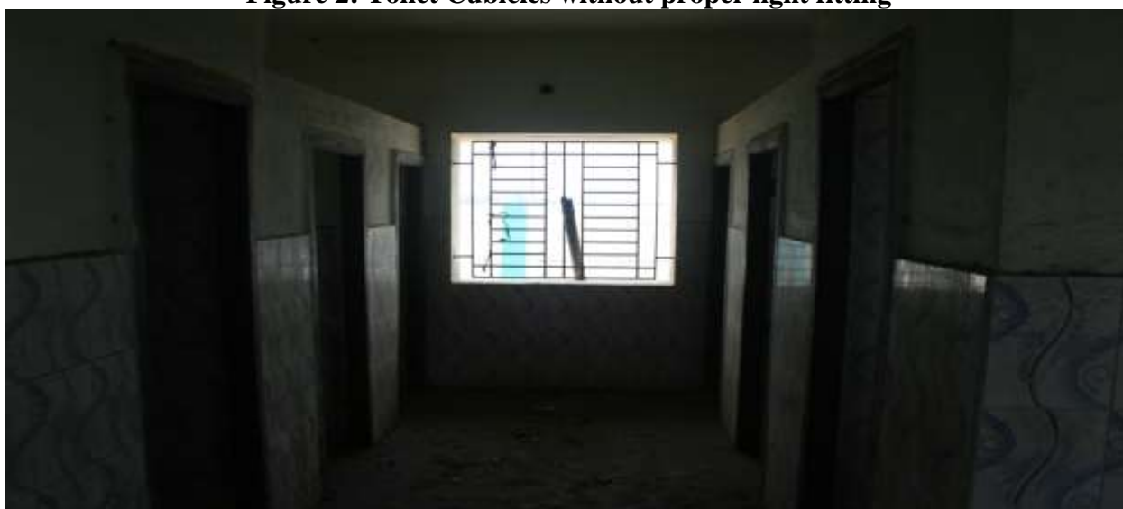
Figure 2: Toilet Cubicles without proper light fitting
