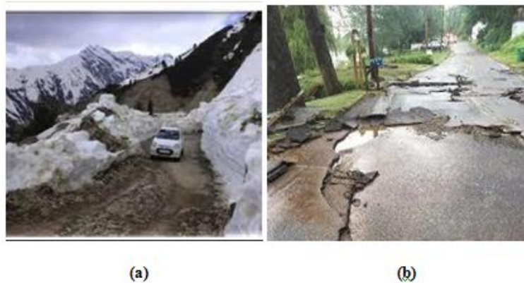
Fig. 2 Deteriorated condition of road (a) due to heavy snow fall (b) because of floods
