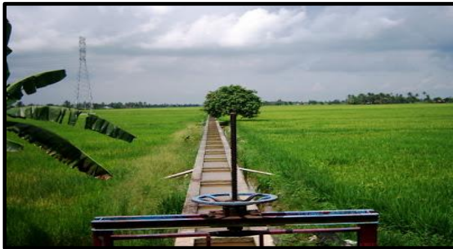
Figure 1 : Water Ropes Or Water Trunks Were Built To Carry River Water To Paddy Fields
