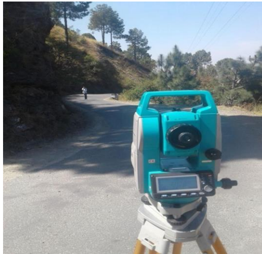
Fig 3- Field surveying via Total Station at Jaswantdwar
