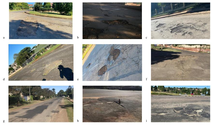
**Figure 9**: Road riddled with potholes (a - f) and the good to poorly repaired roads (g - i)
