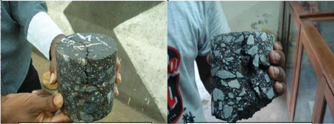
Fig. 6 Core from Km 45.300 32.350 Chennai-Tada road, N.H.5
