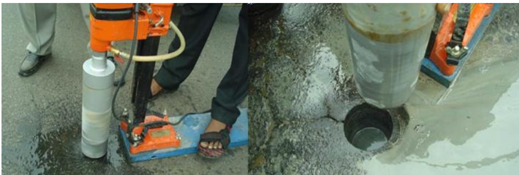
Fig. 5 Core cutting in progress Km 32.350 Chennai-Tada road, N.H.5
