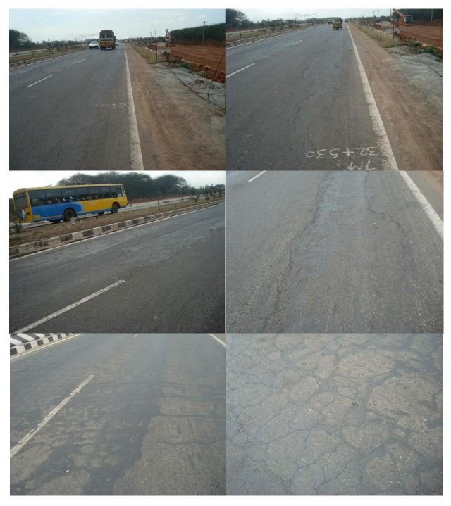
Figure 2: Severe wheel path fatigues cracking, rutting, shoving, and inadequate cross slope Chennai-Tada Road NH-5.
