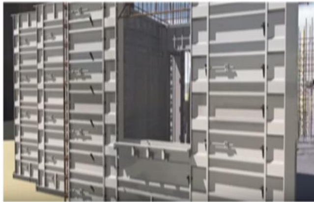
Figure 5. Placing of formwork
