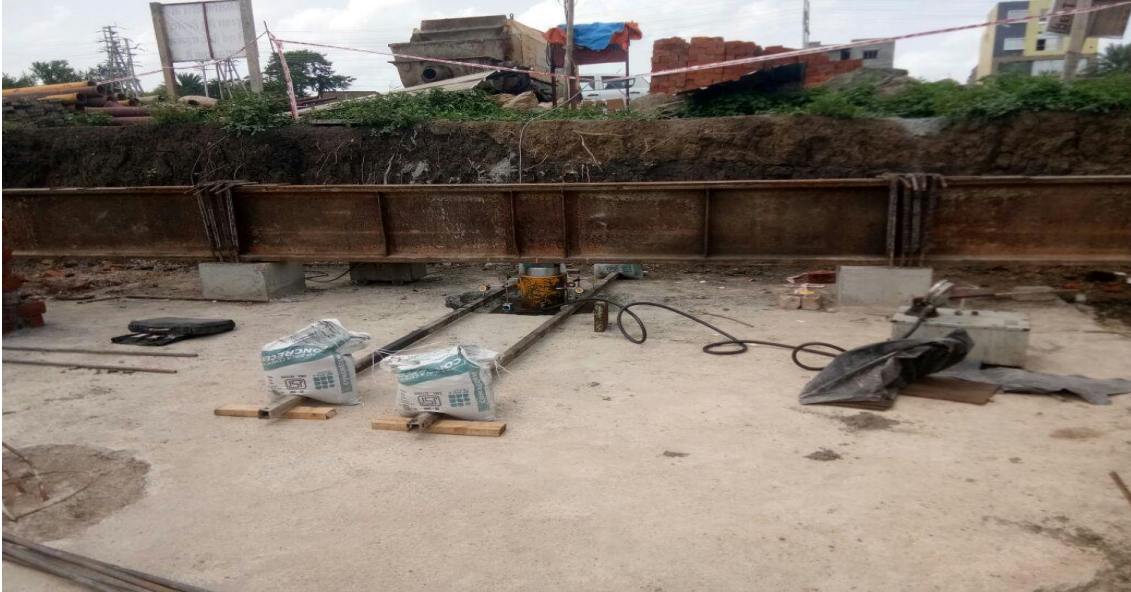
Figure 4: Pile loaded beam with jack application
