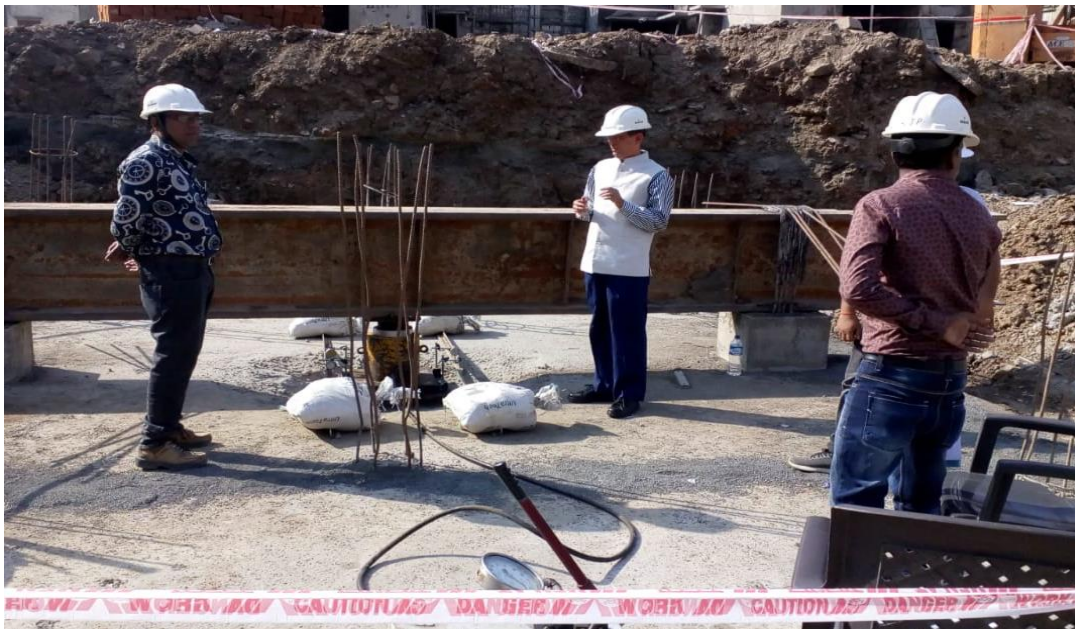
Figure 3: Pile loaded at site
