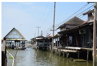
Figure 2: The front of the house, next to the waterfront walkway
