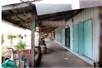
Figure 3: The width of the walkway was approximately 2.50-3.00 m.
