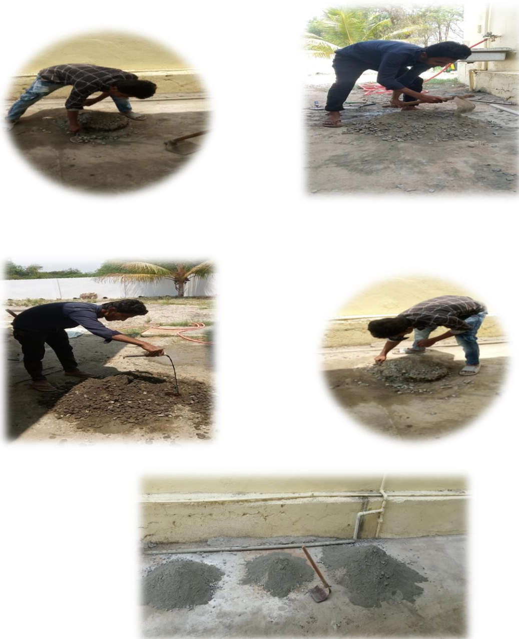
Fig: 3.4. concrete mixing progress
