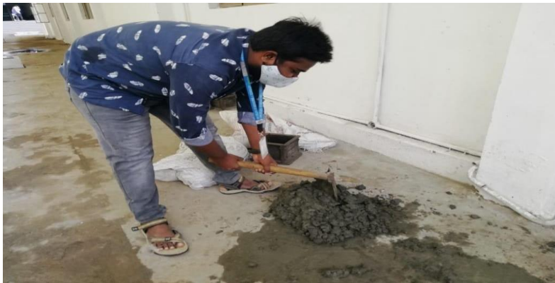
FIG-2.6. MIXING OF CONCRETE
