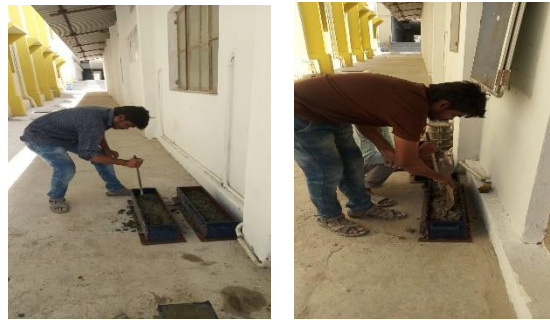
Fig 3.4 Casting of beams
