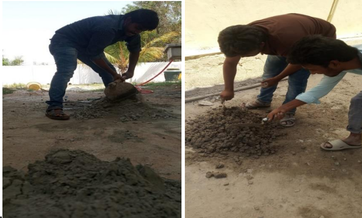
Fig 3.2 Mixing of concrete
