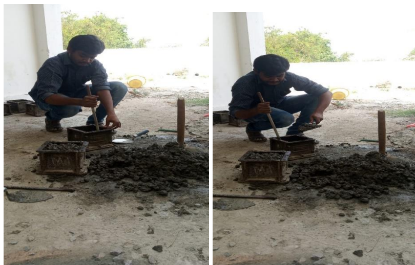
Fig 3.3 Casting of cubes
