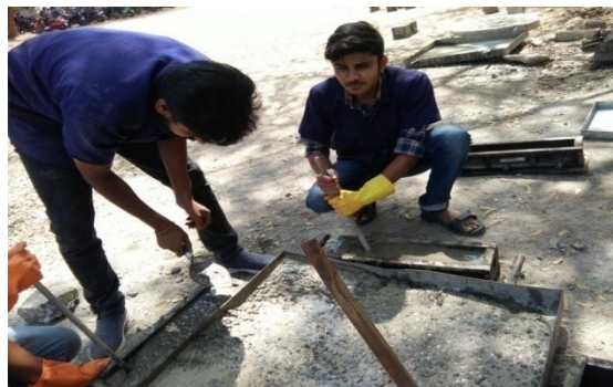
Figure 3.2 Compaction of prism mould
