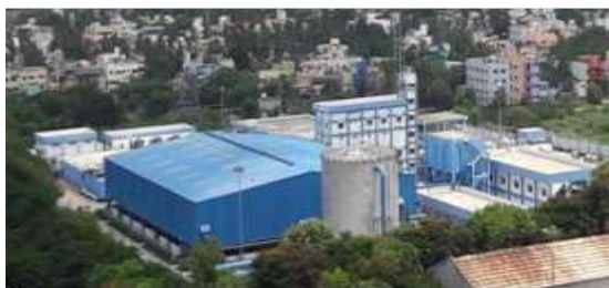
Fig.10.The recent 40 MLD tertiary treatment and advanced filters and membranes buildings
