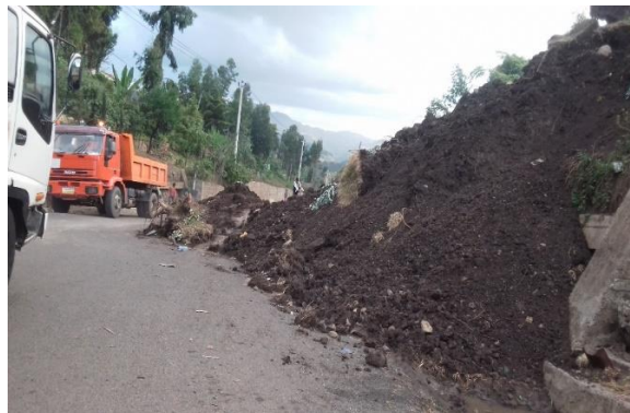
Fig. 5. Failure of earth slope covered almost half of the existing Kombolcha to Dessie Road
