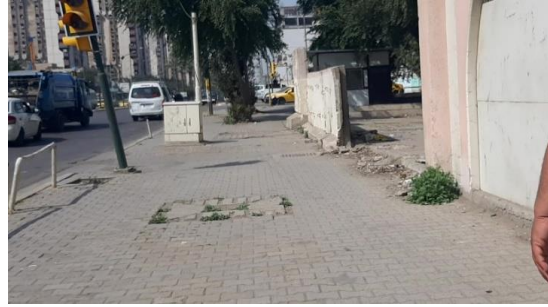
Figure 28. The intersection of Al-Nasr Street with Haifa Street
