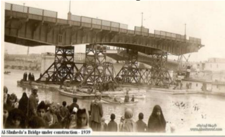
Figure 10. Al- Shuhada Bridge is under construction 1939.
