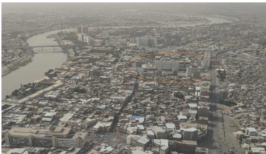
Figure 1. Al-Maidan Square and Surrounding Streets case study- 2020, Google Earth.
