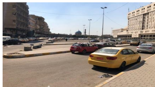
Figure 6 shows Al-Ahmadi Mosque in Al-Maidan Square at 2020 AD / source the researcher
